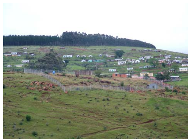
Figure 1 Upper Mnyameni (Treatment Plant in Foreground Enclosure)
