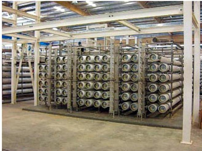
Figure 15: Example of encased membrane
