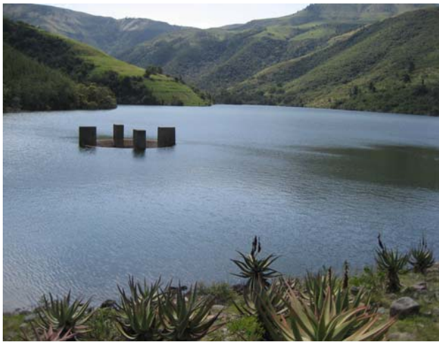
Figure 5. The Upper Mnyameni Dam.
